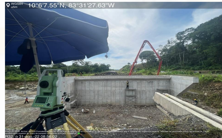
Paso Superior Vehicular Km 95+212
