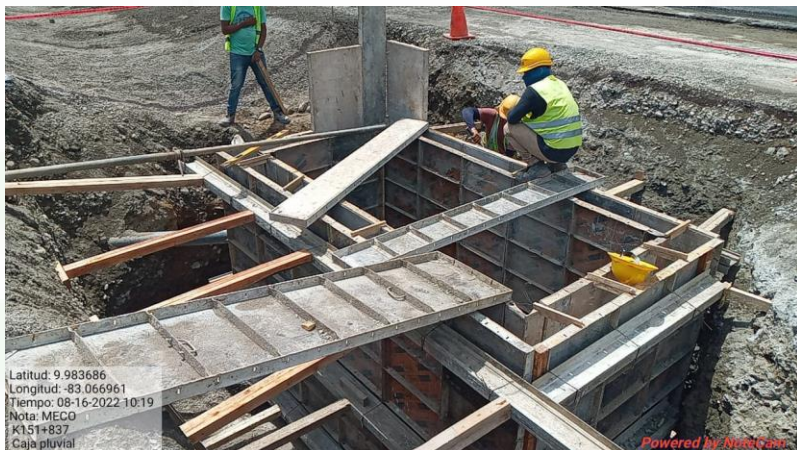
Alcantarilla tubular de concreto Km 151+837, Lado central
