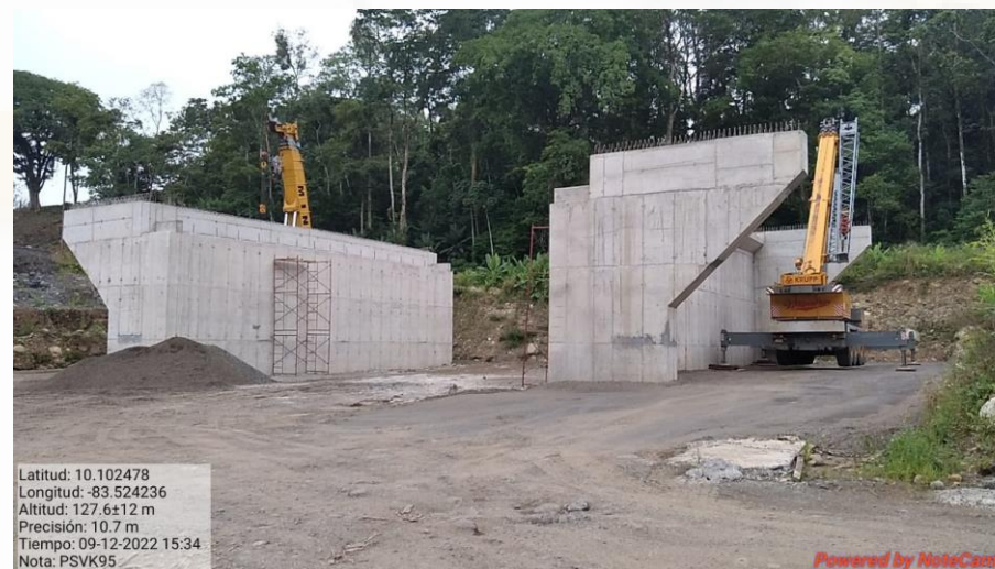
Paso Superior Vehicular Km 95+212
