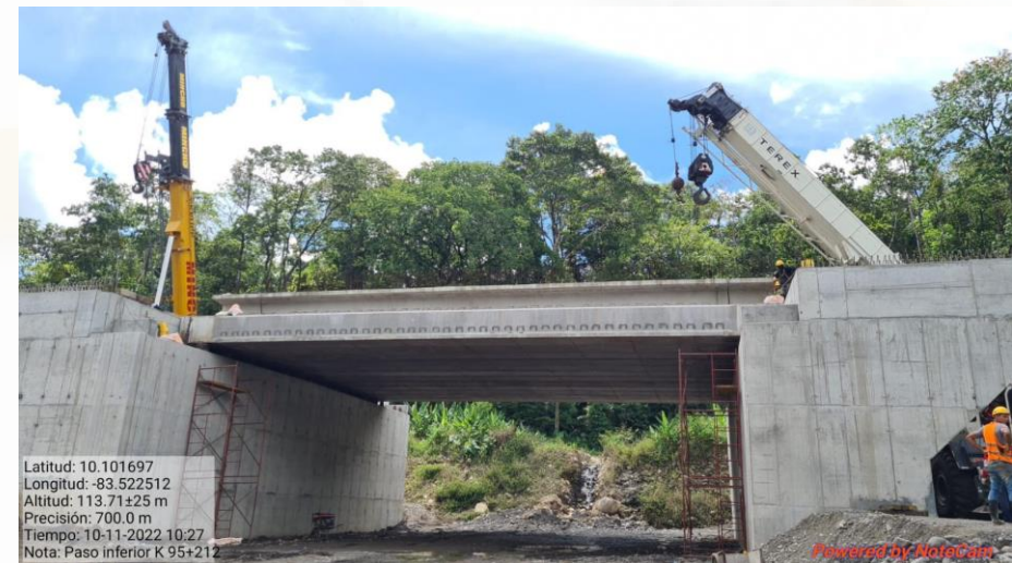
Paso Superior Vehicular Km 95+212
