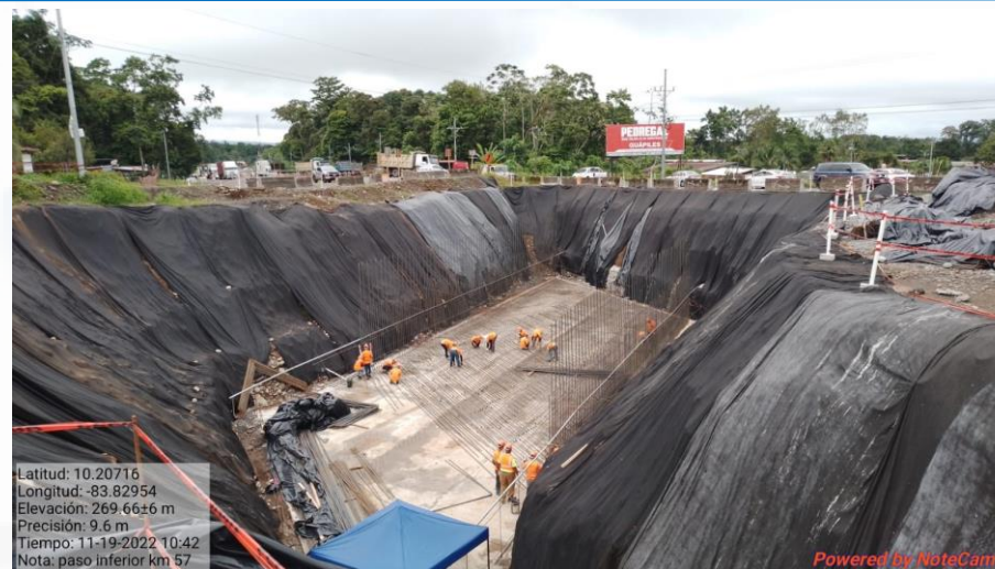
Paso Superior Vehicular Km 57+533
