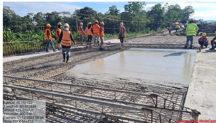
Paso Superior Vehicular Km 95+212
